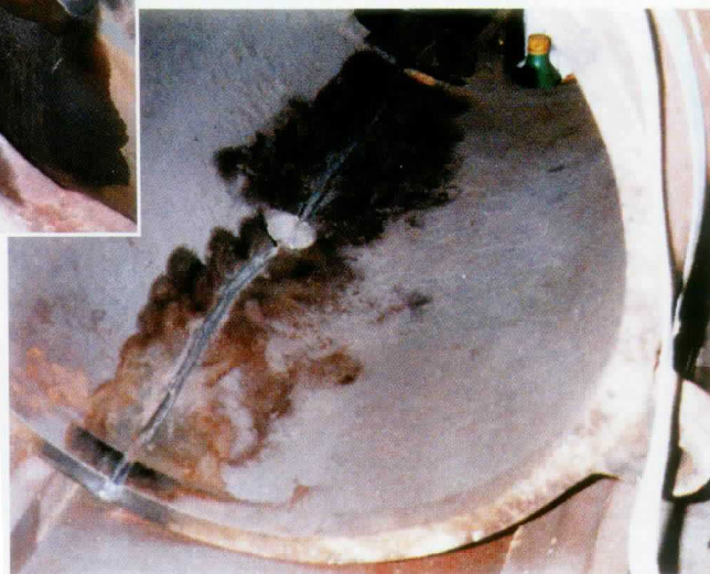
Below: Freeze crack ran the entire length of the cylinder water jacket.
